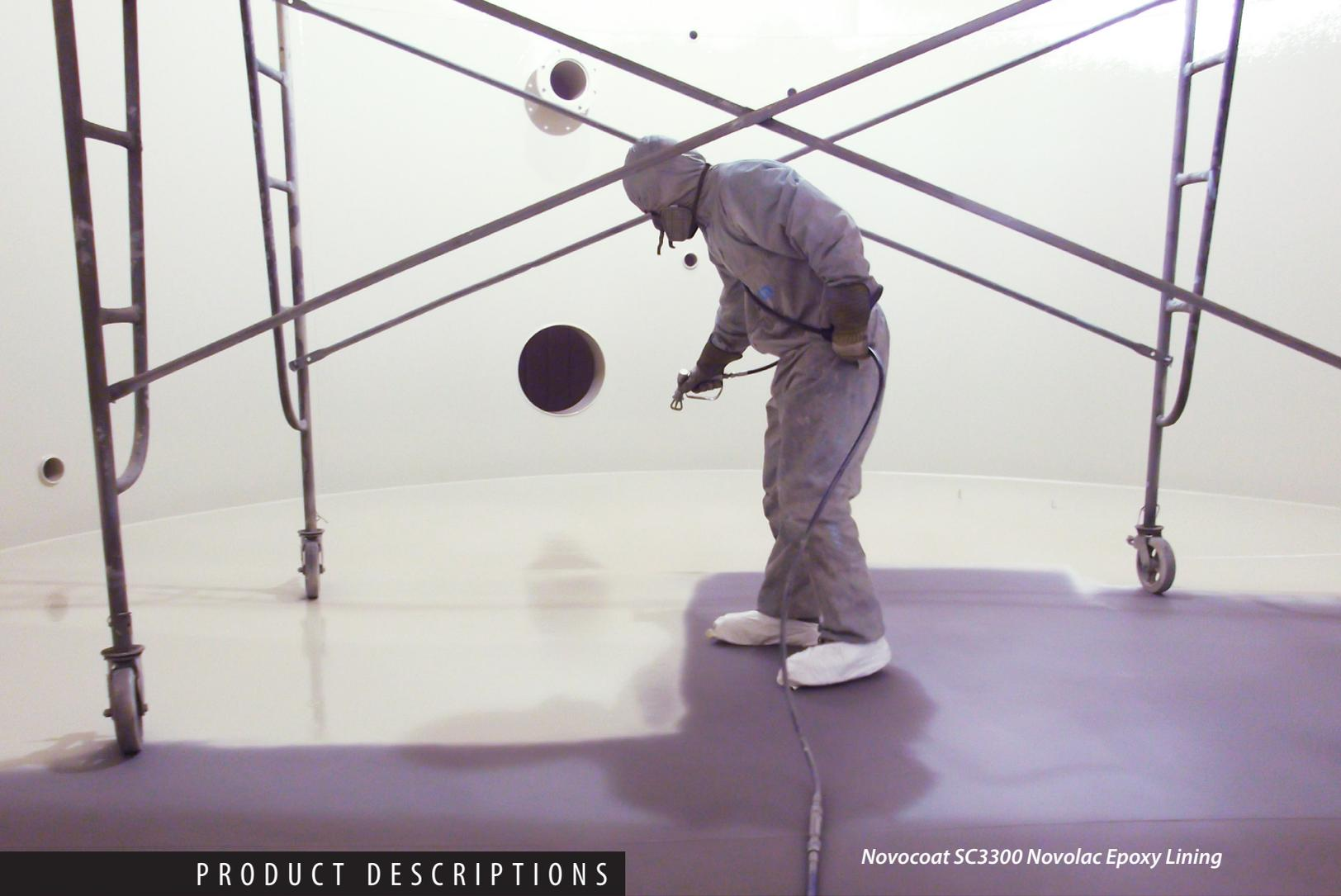
*Novocoat SC3300 Novolac Epoxy Lining*
